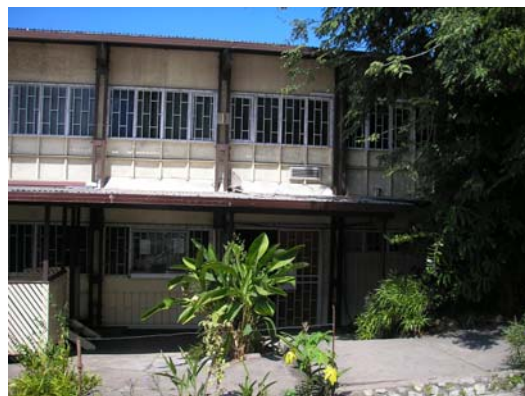
Lands Commissions' Office, Four Mile, Port Moresby. Record Room on Right, below.
