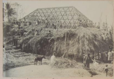
Putting the roof on Epi
