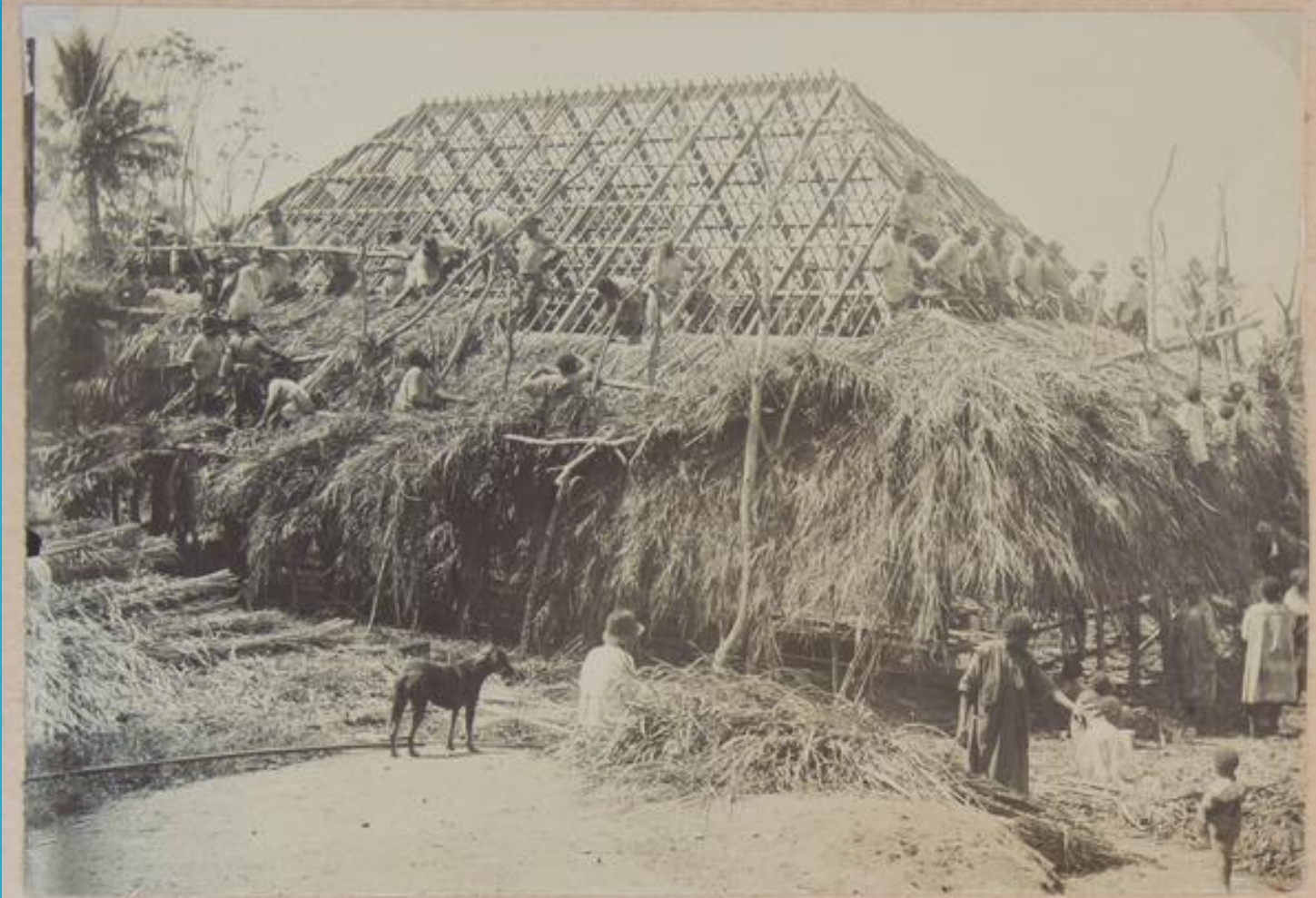
Putting the roof on Epi
